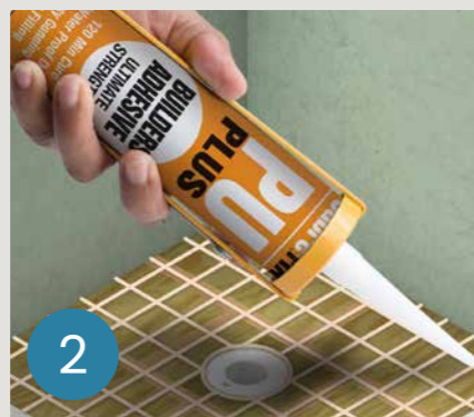
2 Applying polyurethane adhesive
