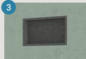
3 Install niche, ensuring front face is flush with front face of Gib/Villa Board.
