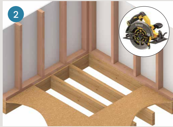
2 Cut out 20mm flooring and remove.
