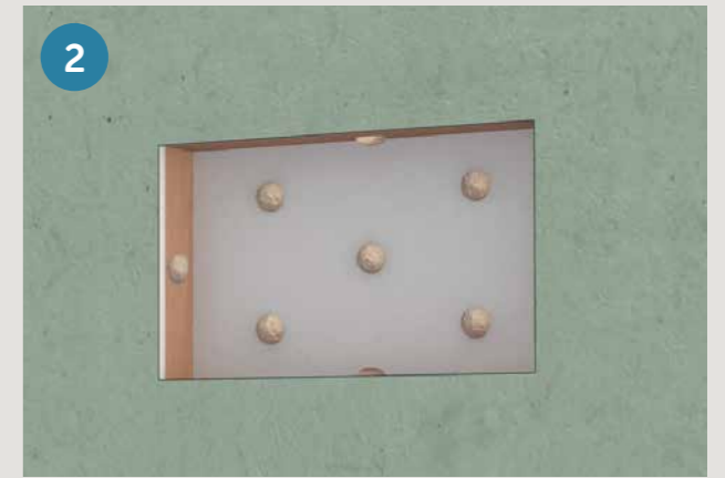
2 Fix Gib / Villa Board, dry fit niche, remove and apply adhesive.
